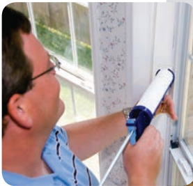
Caulking along moldings and joints with a sealant.
